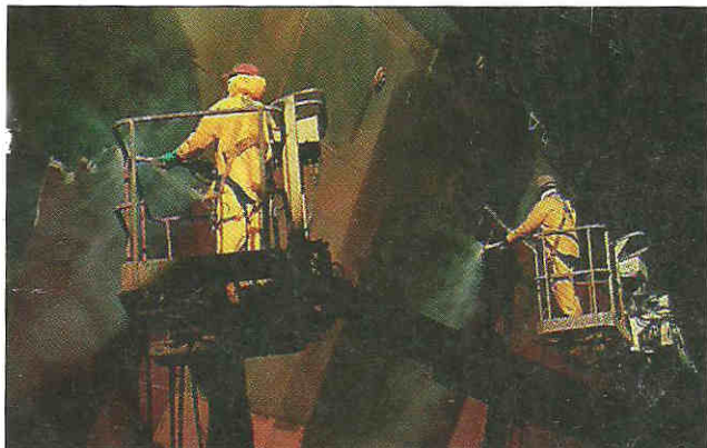
Ultra high pressure water jetting at Todd Pacific Shipyards, Seattle (p. 22)
