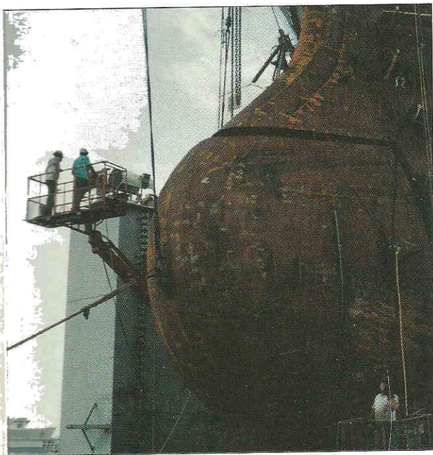
On our cover: Repairs to the Alexia at Bender Shipbuilding & Repair, Mobile, Alabama (p. 21)
