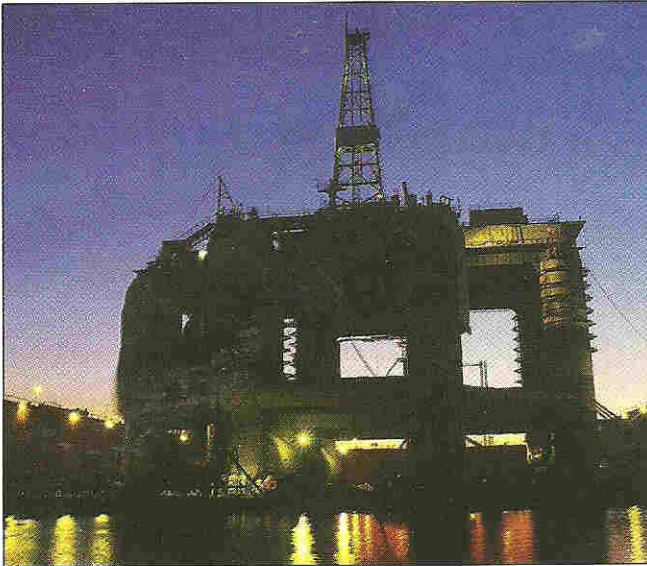
This month's cover shows the offshore rig Ocean Quest at Texas Drydock, Inc. as it nears completion of upgrading for deeper water operations (p. 25)
