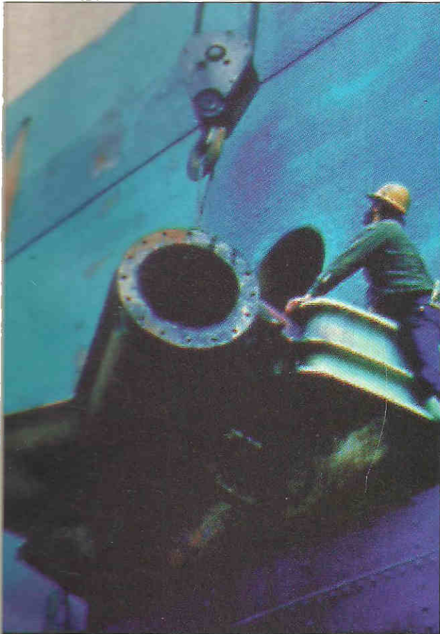
Cover photo shows removal of the old condenser water box from a foreign-flag cruise ship at Norshipco, Norfolk, Va., prior to fitting new equipment fabricated before arrival of the vessel. U.S. ship repairers continue to report an increase in commercial ship work (p.25)
